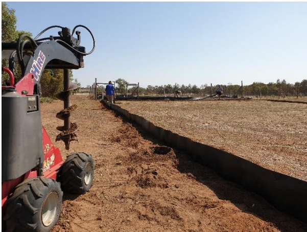
Figure 2 drilling holes for posts
